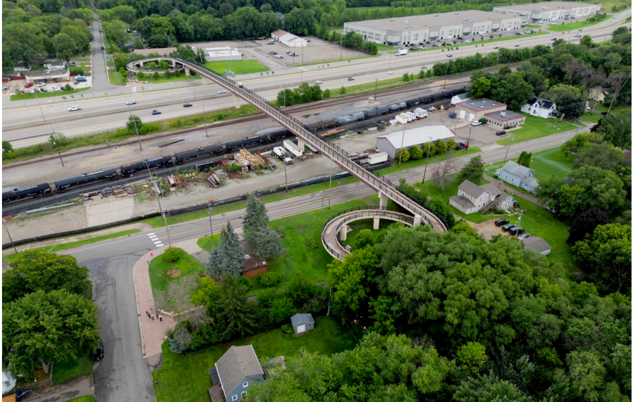
Figure 5: Bridge for people walking and biking in St. Paul Park.
